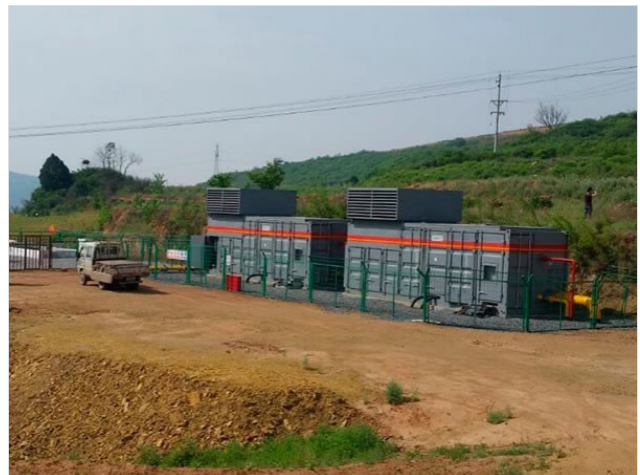
Coalbed methane compressors for Asian American Gas Inc 70000M3/D 320KW 380V motor driven 100000M3/D 420KW 6000V motor driven
