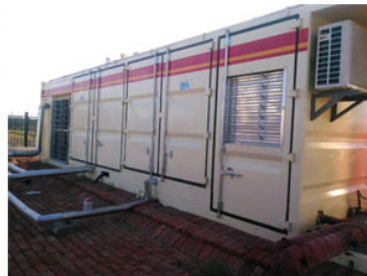
Skid integrated CNG compressor,with interstage dry dehydration system Suction pressure 0.15MPa,discharge pressure 25MPa,10,000Nm3/Day
